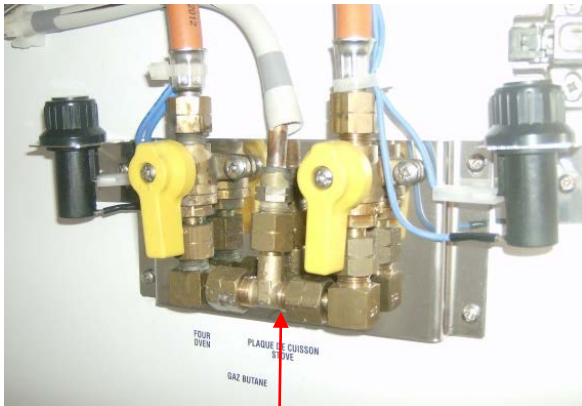
Gas shut off valves under sink
