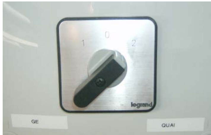
Generator (GE) / Shore power (QUAI) selector switch
