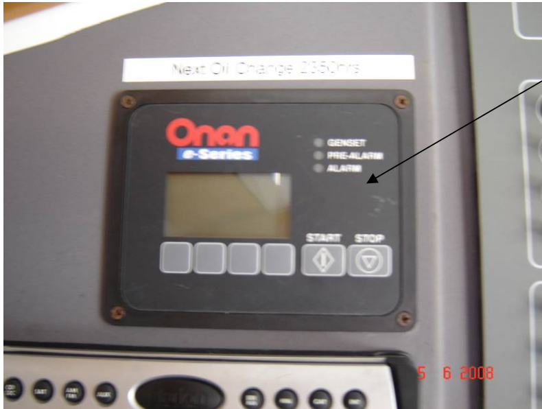
Generator panel for starting and stopping the generator
