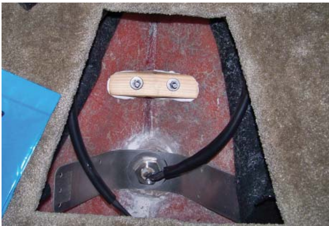
Fig. 36: boat interior bolting GRP
