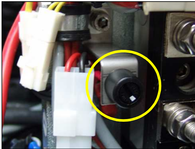
Fig. A.3.5-11: Fuse for Measurement Voltage
