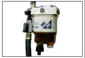
Fig. B.5.3-1: Fuel filter with water separator
