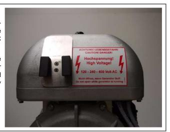
Fig. A.4.6-5: Generator power terminal box
