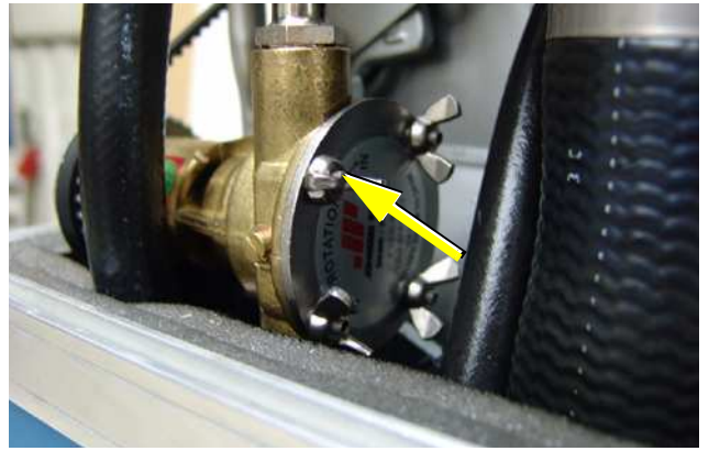
Fig. C.7.3-3: wing screw raw water pump
