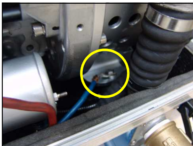
Fig. C.7.1-2: Negative battery cable
