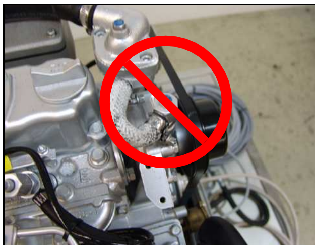
Fig. E.5-4: Ventilation screw above the cooling water pump casing
