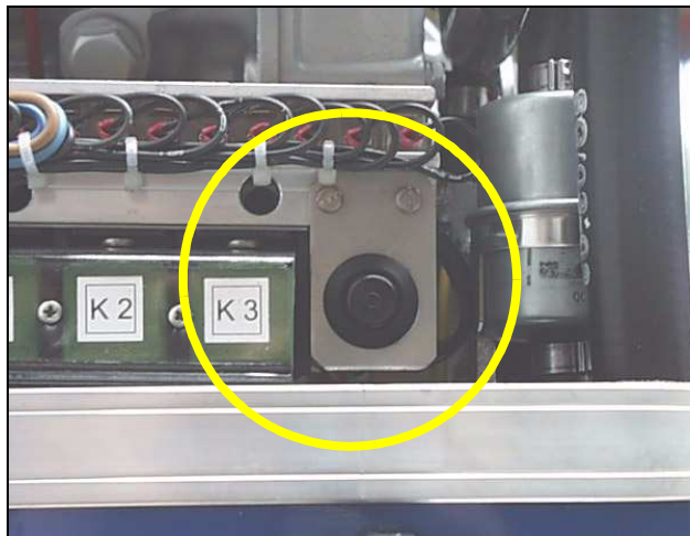
Fig. A.3.6-6: Failure Bypass switch
