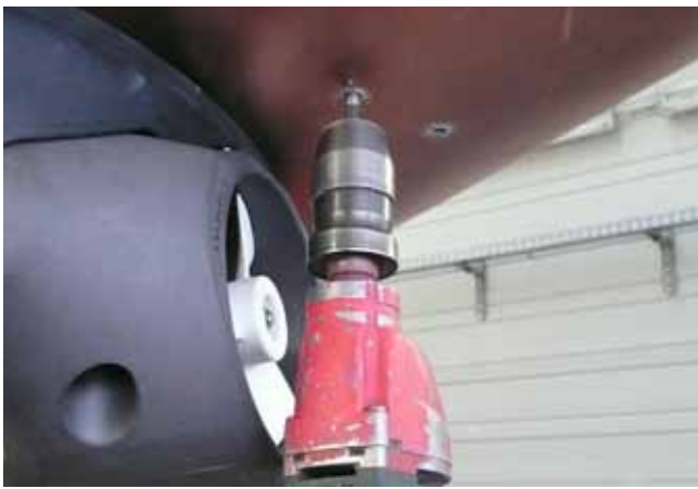
Fig. 19: mounting bolts drilling
