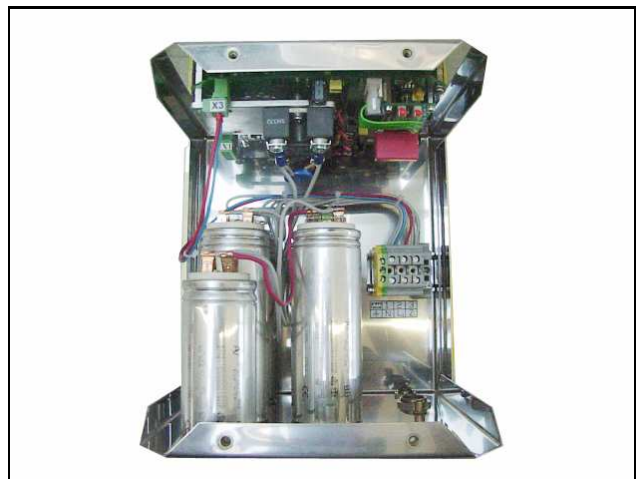
Fig. A.3.8-2: Opened AC Control Box
