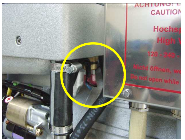
Fig. A.3.6-2: Thermo Switch at Water Cooled Exhaust Elbow
