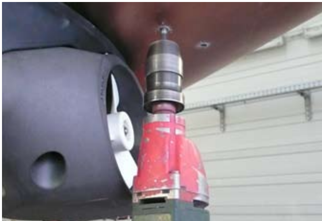
Fig. 19: mounting bolts drilling
