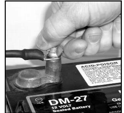
Figure 6 - Mounting temperature sensor on battery negative terminal post.
